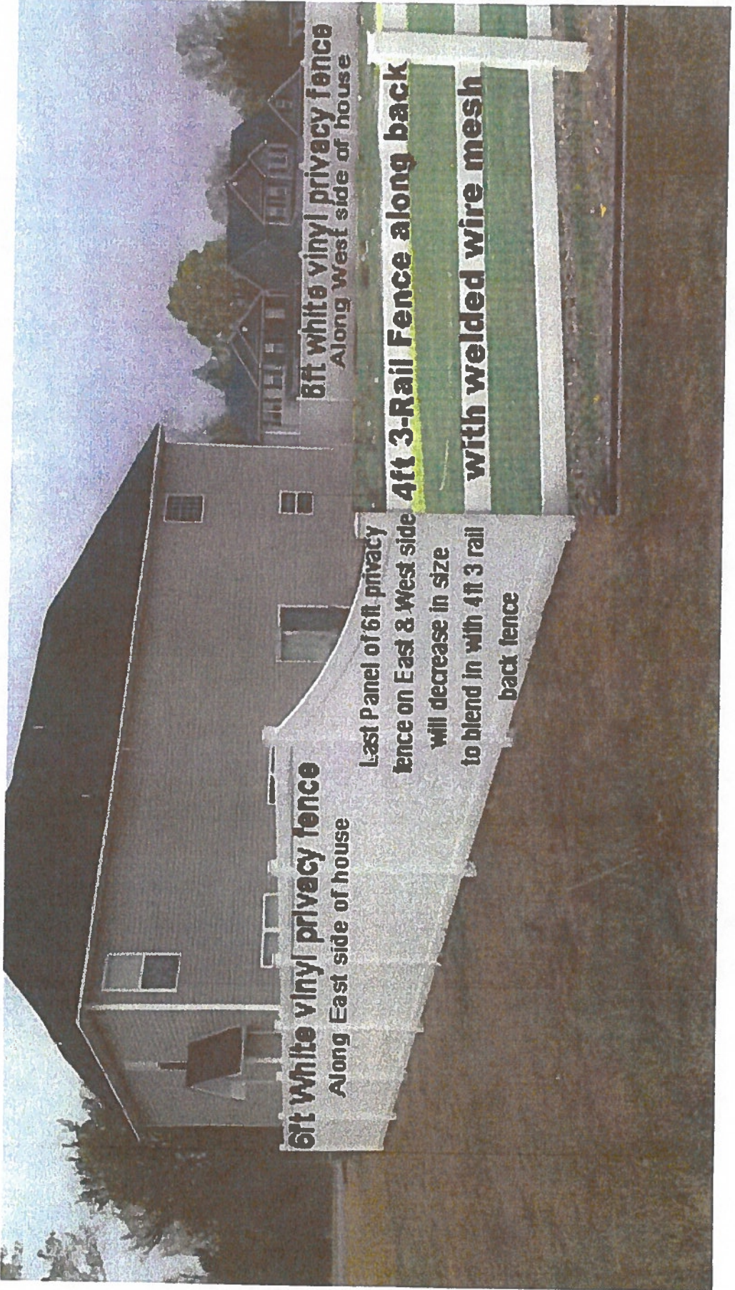
Example of sloped fencing when connecting privacy fence to three rail fence.
